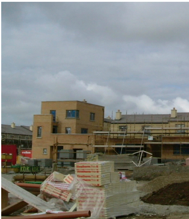
Tyrrelstown Housing, Dublin, Irsko
