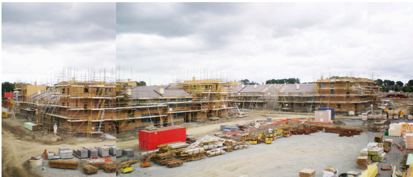
Tyrrelstown Housing, Dublin, Irsko
